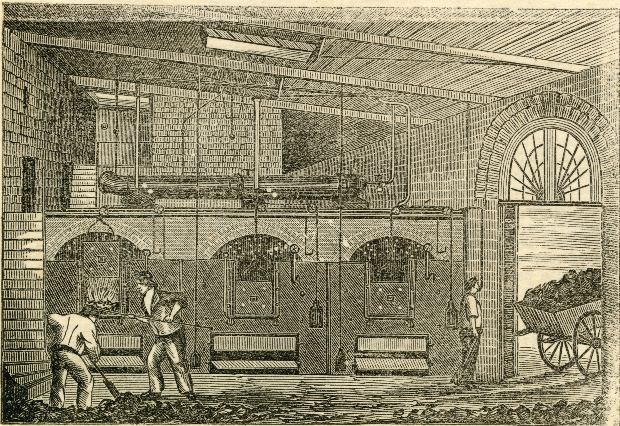
No. 1.—BOILER HOUSE.
