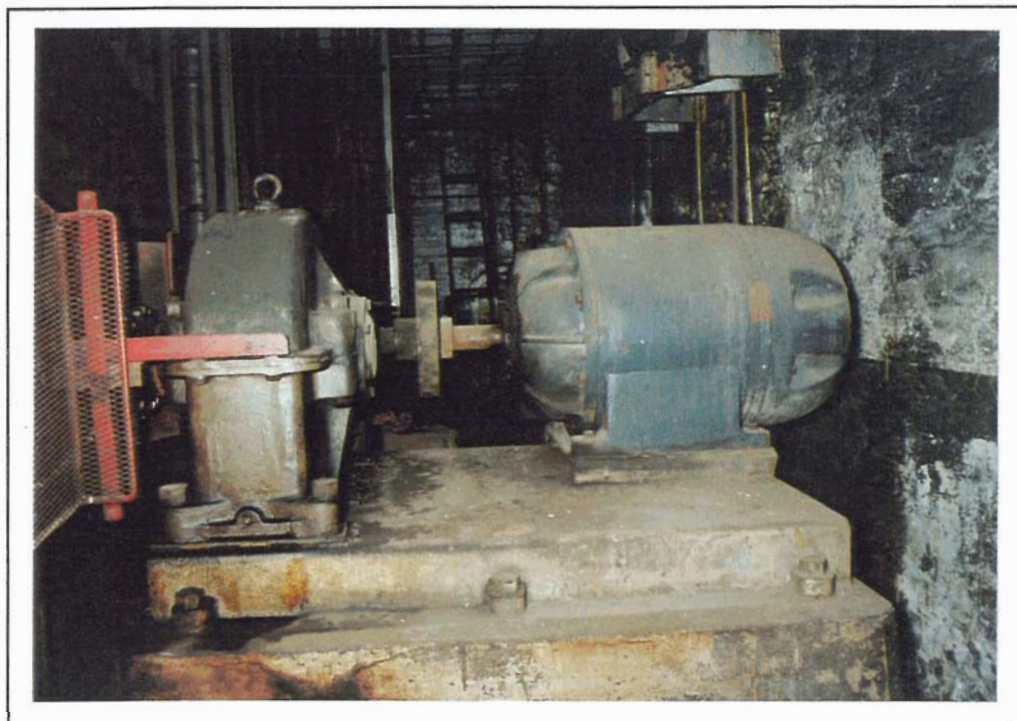
5A-1-2 Motor and Transfer Case
