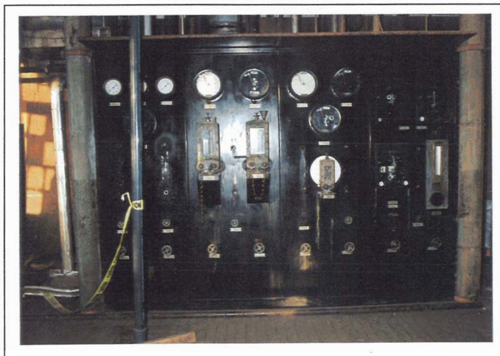
5-2-10 Distillation Control Panel
