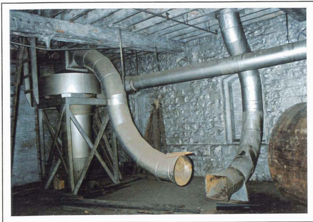
4-4-4 Grain Hopper/Blower with Ducts
