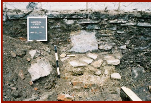
Foundation abutting Building 31
