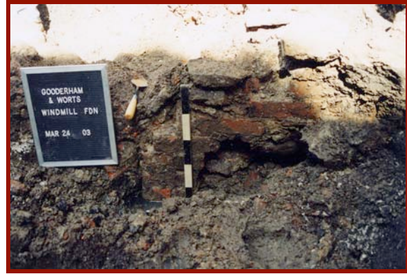
Close-up of brick arch in foundation
