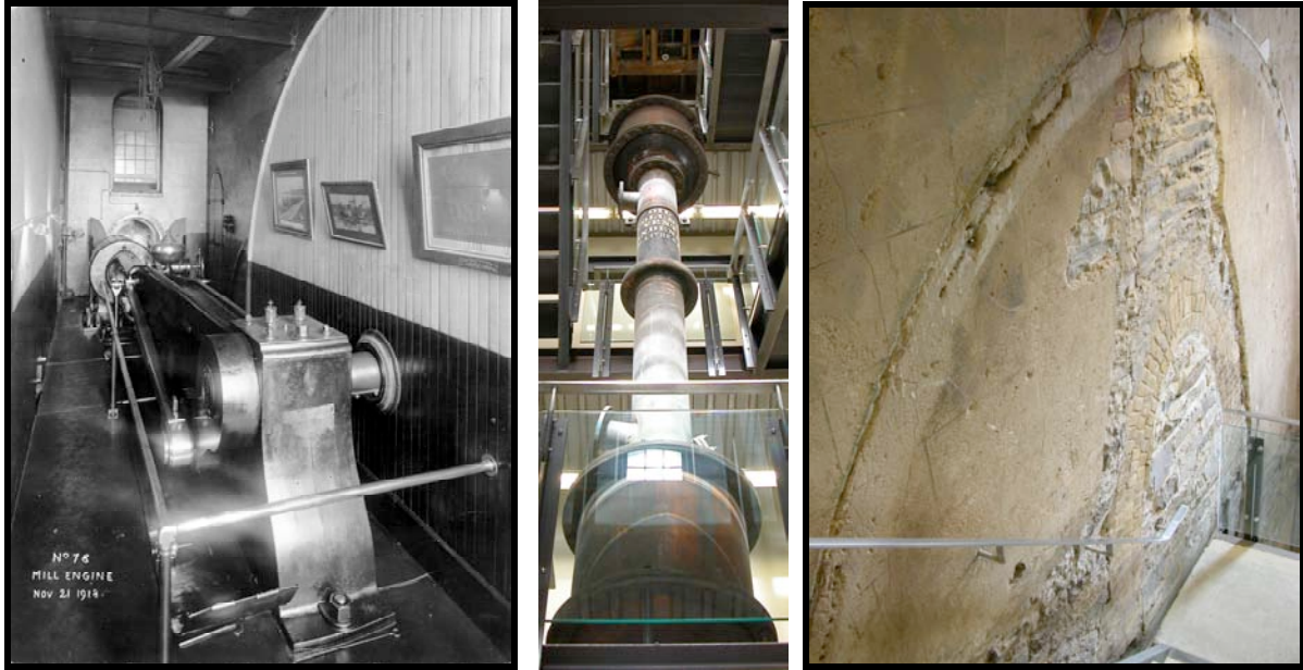
Engine Room, 1918 CTA Stairwell 2007 Outline of Flywheel Housing
